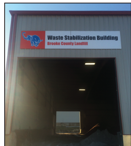
Wet drilling waste stabilization building.
